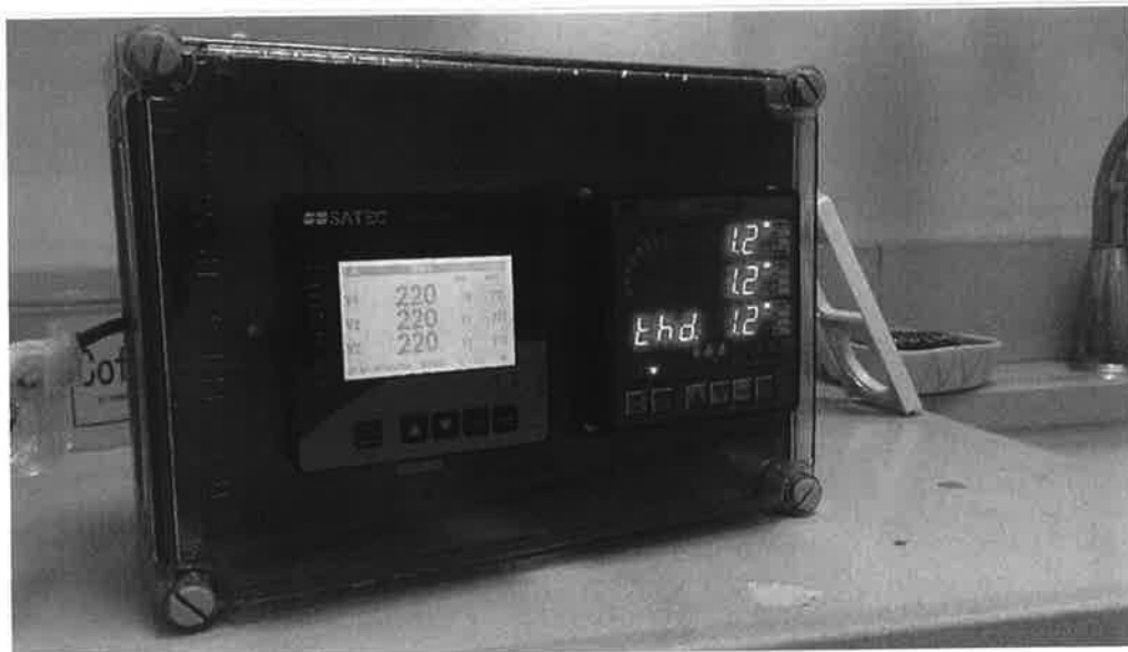
Figure 3.5—UUT after the Water test
