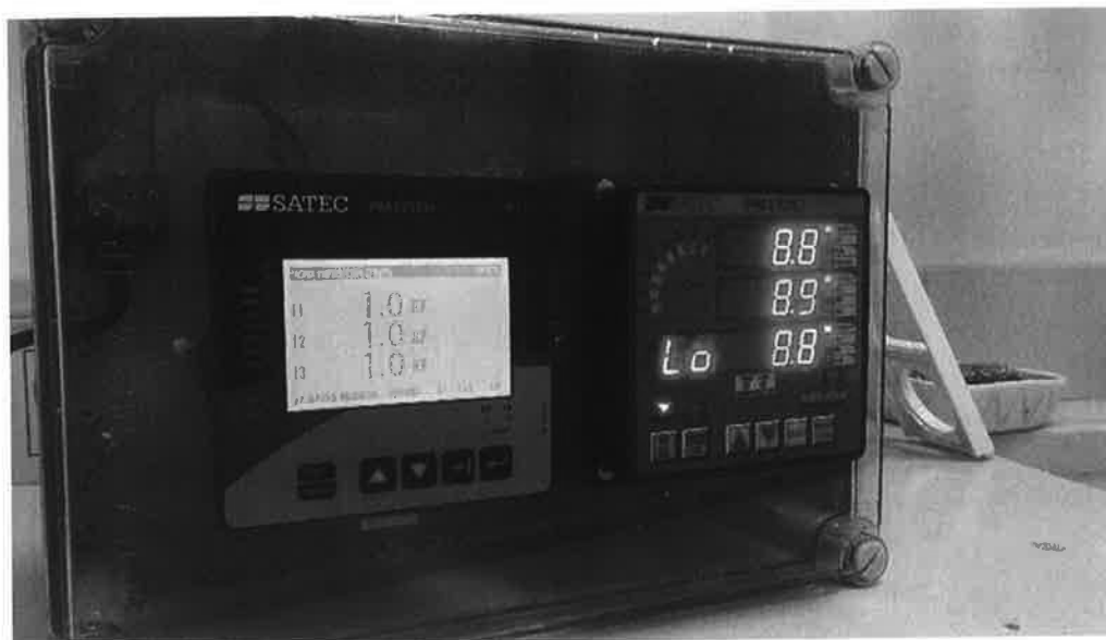
Figure 3.6—UUT after the Water test
