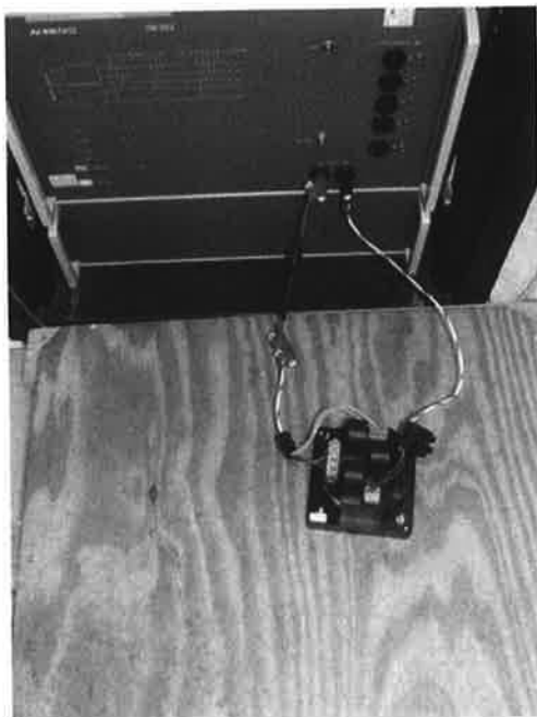
Test Picture 4: Surge on PM130EH Plus
